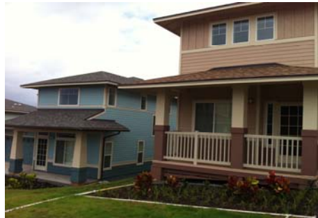
Radar Hill Family Housing
